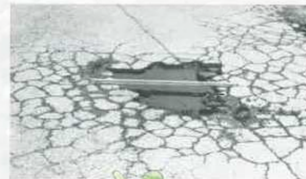
Figure 13c. High-Severity Pothole.
