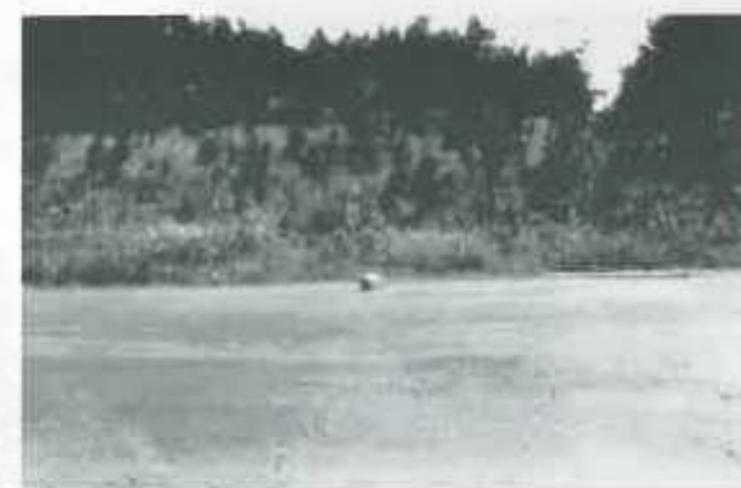
Figure 18. Example Swell. Severity level is based on ride quality criteria.
