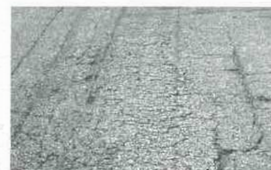
Figure 19b. Medium-Severity Weathering and Raveling.
