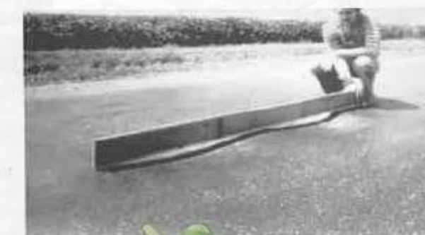
Figure 5c. High-Severity Corrugation.
