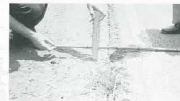
Figure 9b. Medium-Severity Lane/Shoulder Drop-Off.
