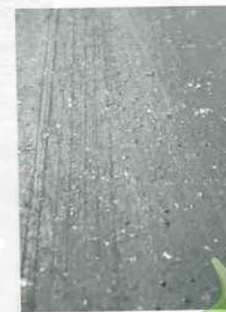
Figure 2c. High-Severity Bleeding.
