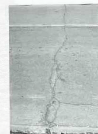
Figure 8b. Medium-Severity Joint Reflection Cracking.
