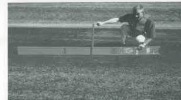
Figure 6a. Low-Severity Depression.
