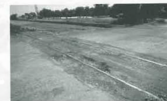
Figure 14c. High-Severity Railroad Crossing.
