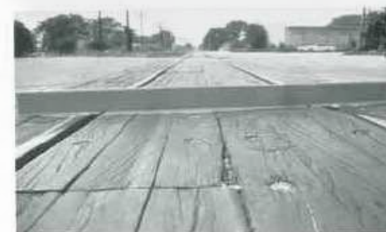
Figure 14a. Low-Severity Railroad Crossing.
