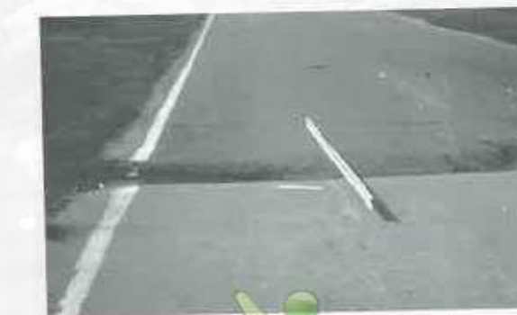
Figure 16c. High-Severity Shoving.
