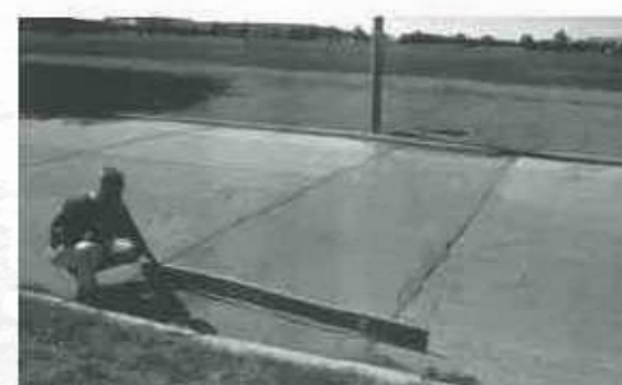
Figure 11b. Medium-Severity Patching and Utility Cut Patching.
