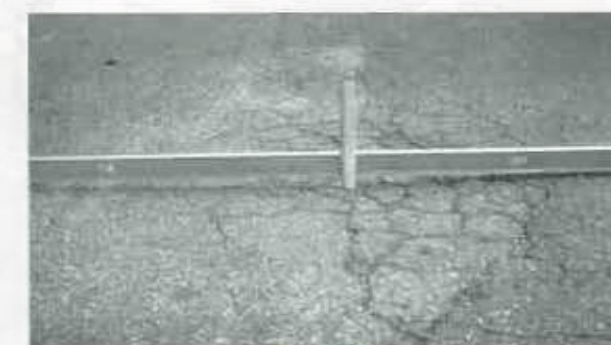
Figure 6c. High-Severity Depression.
