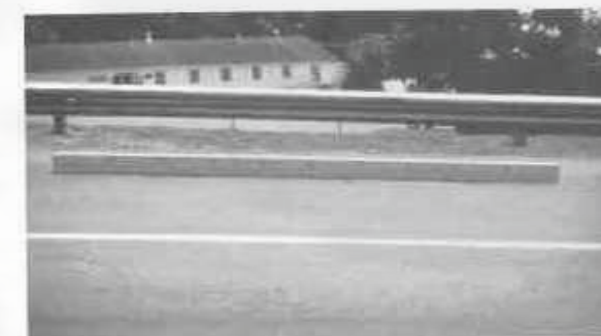
Figure 5a. Low-Severity Corrugation.
