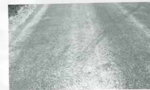
Figure 2a. Low-Severity Bleeding.
