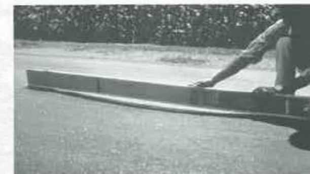
Figure 6b. Medium-Severity Depression.
